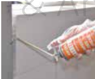
Thin vertical/horizon. joint sealing
