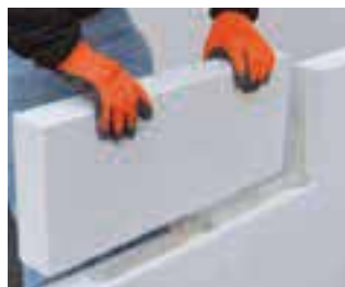
GASBETON® block laying
