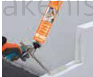
GASBETON® block laying
